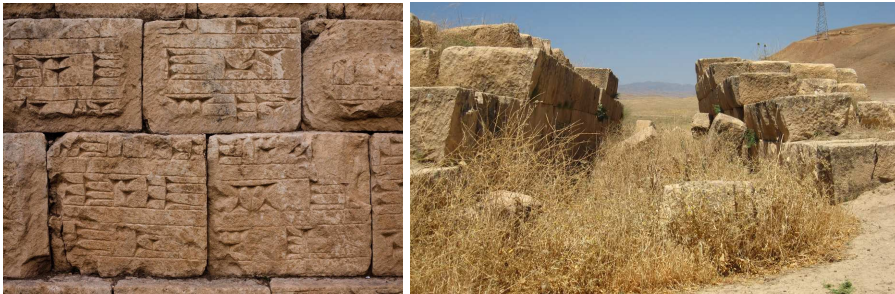
Fig. 10. Left – The cuneiform inscriptions on the stone blocks used for construction of the Jerwan Bridge structure, preserved to this day [W16]. Right – A current view of one of the corbelled false-arches used in the bridge under consideration [W17]
