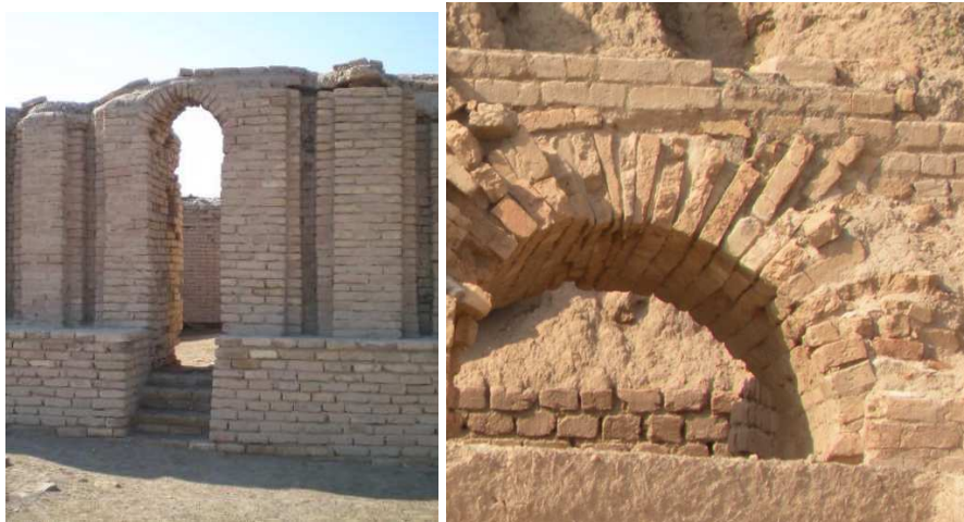
Fig. 3. Left – Partially reconstructed flat „true-arch” brick gate of a small free-span to the Edublalmahr temple in Summerian Ur dating back to 2100 BC [W4], Right – An opening topped with a flat “true-arch” being a part of the Elamite ziggurat in Chogha Zanbil, originating from 1250 BC, reconstructed partially from original brick (photo taken in 2015 by M. Maślak)
