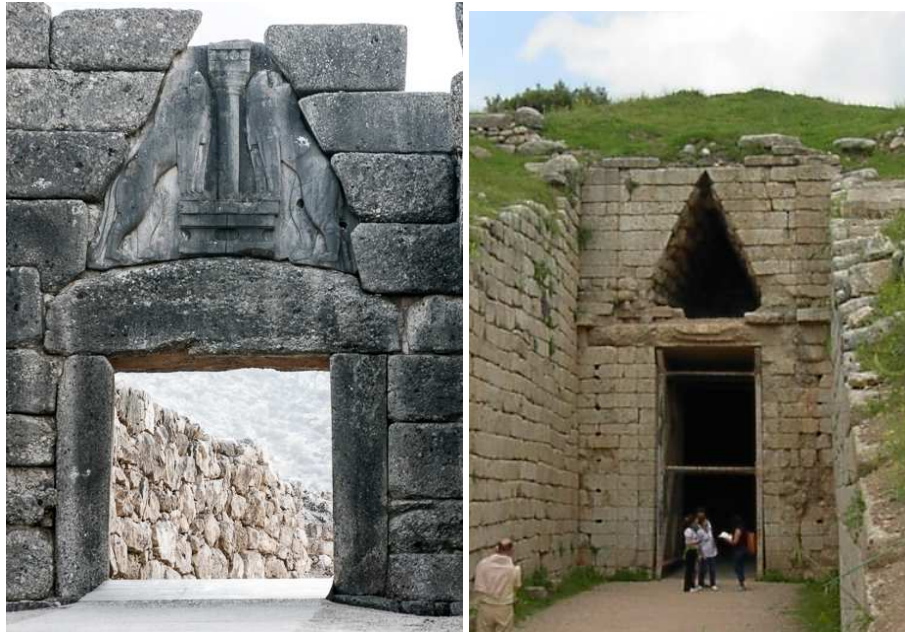
Fig. 5. Left – A corbelled stone false-arch applied in the Lion Gate structure in the citadel of Mycenae in which the massive triangular disc relief the architrave beam [W6]. Left – An analogous triangularly-shaped corbelled stone false-arch used in the entrance to the tholos called the “Treasury of Atreus”, located also in Mycenae but on the Panagitsa Hill, in which the large stone disc is not inserted into the gate structure [W7]
